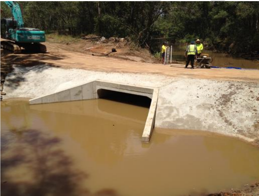
Photo D: Looking at the completed waterway barrier works from a downstream position.
