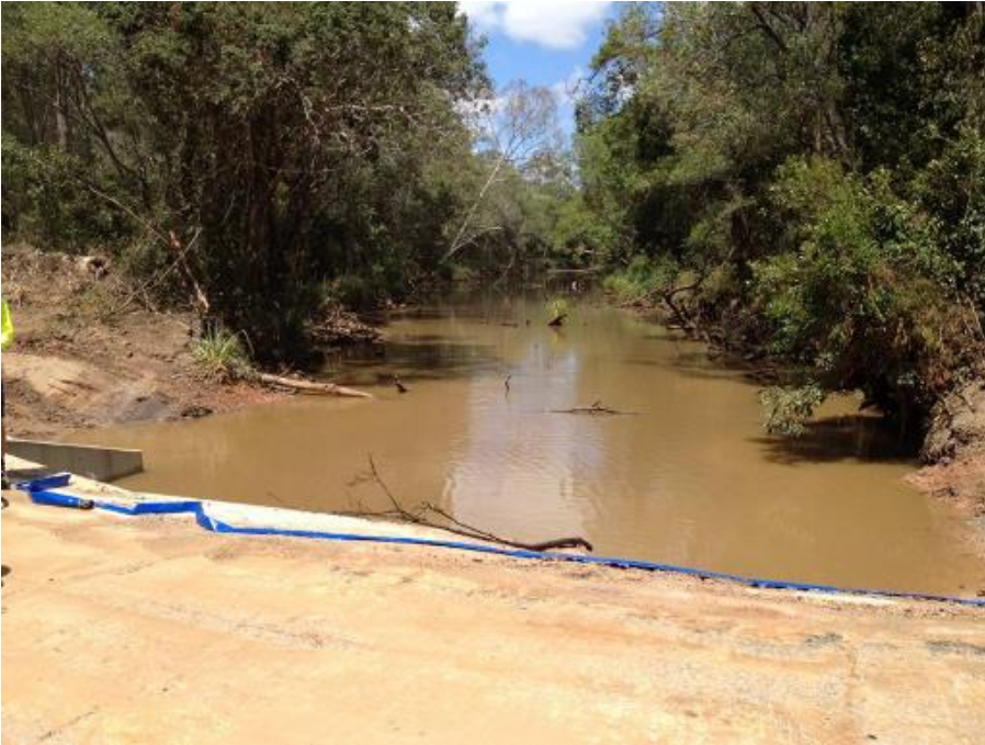
Photo C: Looking upstream (after waterway barrier works).
